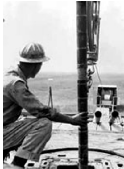
A logging tool about to be lowered into a well
